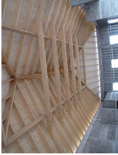
FRAMEWORK WITH ROOFING
